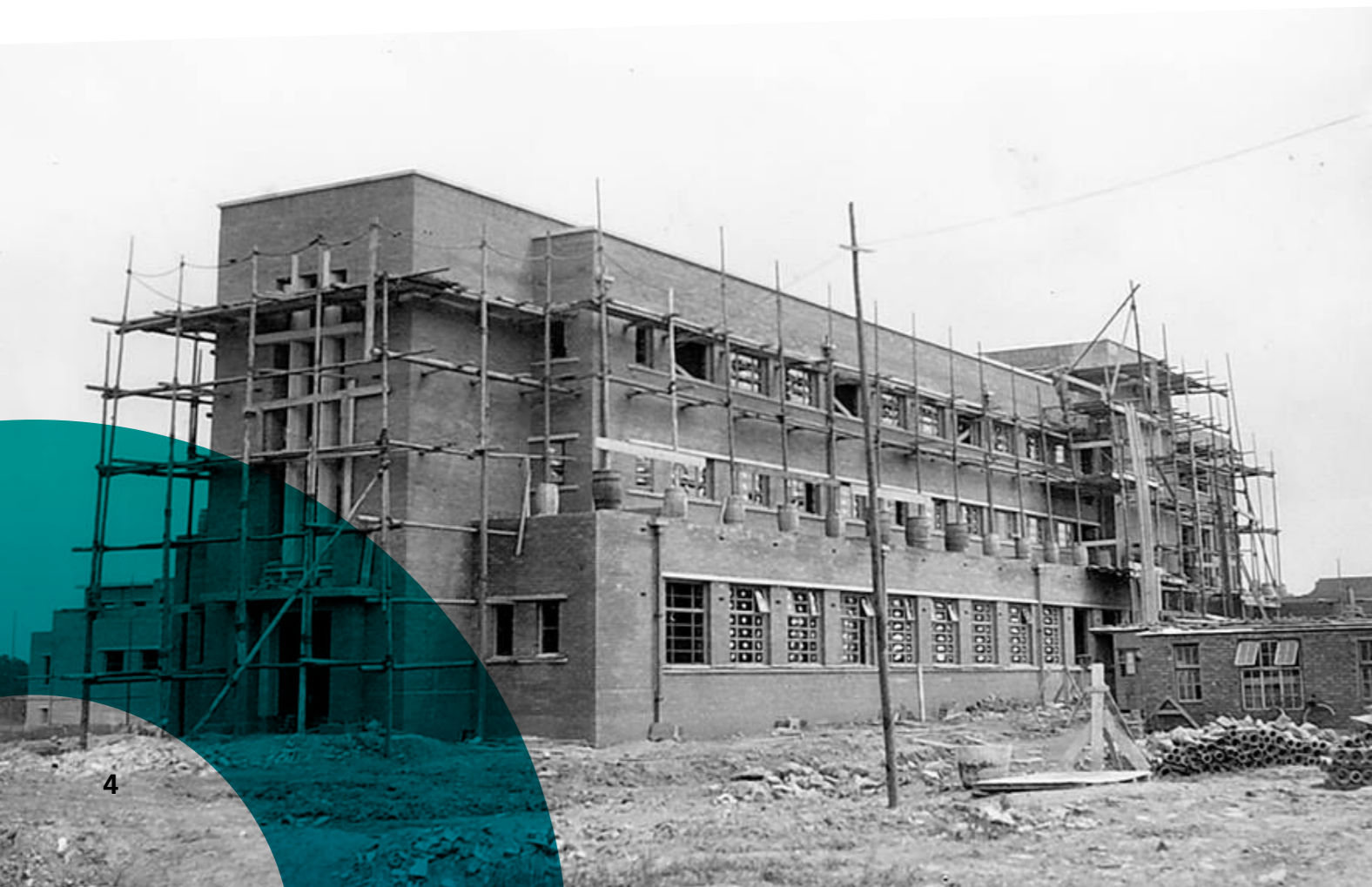
Sunderland Eye Infirmary being built on Queen Alexandra Road, 1939
